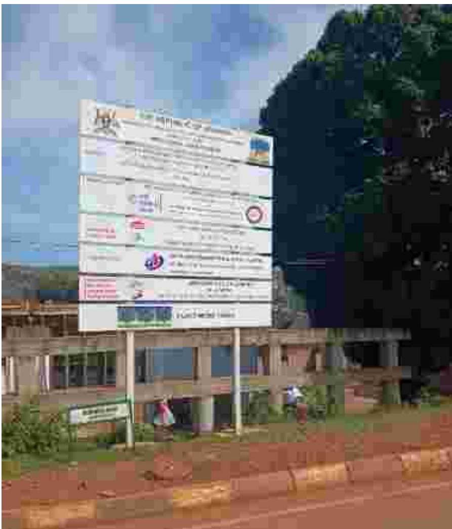
Mpigi-Muduuma Road signage
