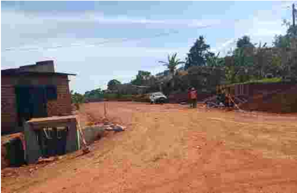
Mpigi-Muduuma Road drainage inlet
