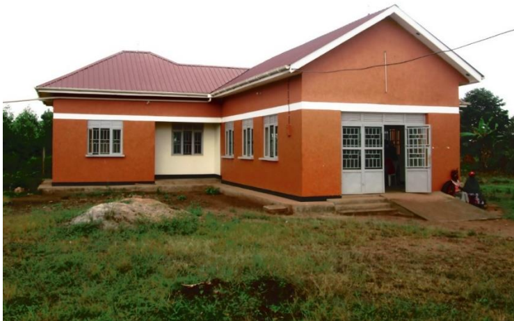
Council Hall with Offices constructed at New Buwama Sub County Headquarters
