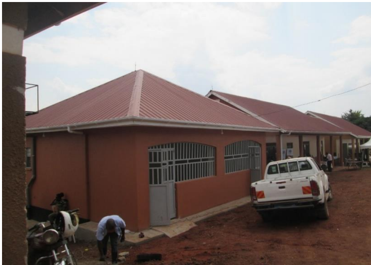
Demonstration structures constructed at the Agricultural Development Centre under DDEG.
