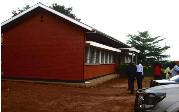
Education and Sports office block after general renovations
